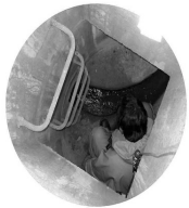
inside the pipe
