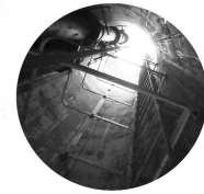
inside strovolos tower 2 .jpg
