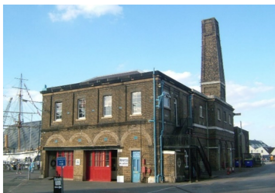
Εικ. 2.41 South Dock Pumping Station (1822).
