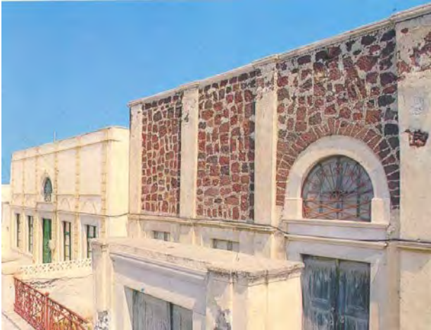
Figure 13, 14. Views of the densely built Oia, with the so-called captain's houses, where the neoclassical elements were mainly confined to the design of the facades.
