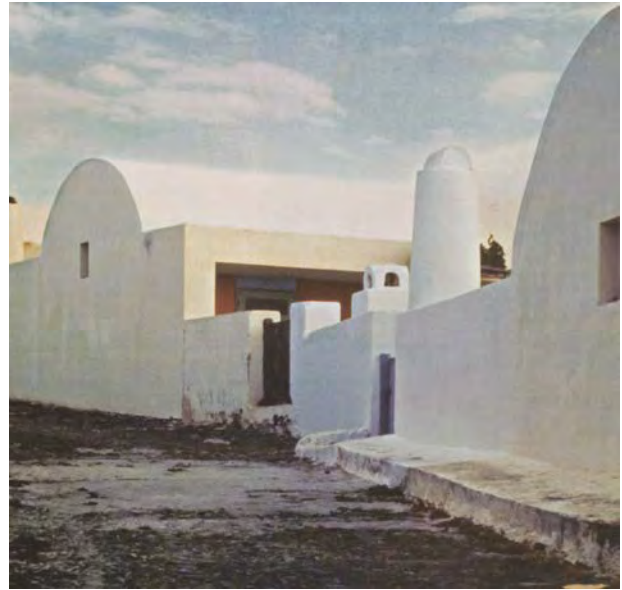
Figure 15. Post- earthquake housing, chief planner and architect C. Decavalla (Design-construction: 1956-60
