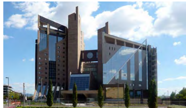
Figure 3. Florence - The New Palace of Justice. The complex is characterised by both local and global design conception and is of a huge appearance impact on the site but with no suitable adaptation to the local environmental and micro climate. (Photo by D. Babalis)
