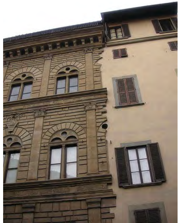
Figure 10. Alberti froze the transformation of row houses into a palace by leaving one of the houses uncovered by the new facade.
