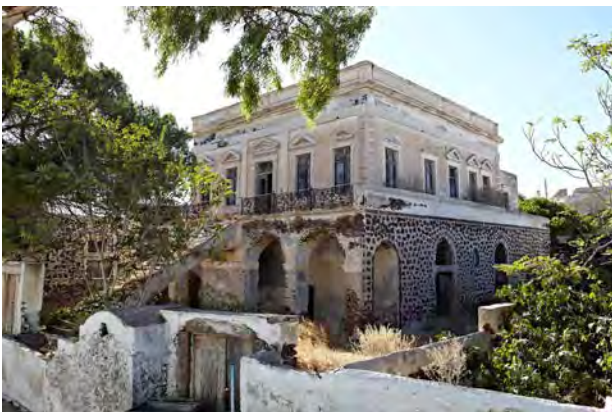
Figure 5. Photo of a Mansion in Massaria.
